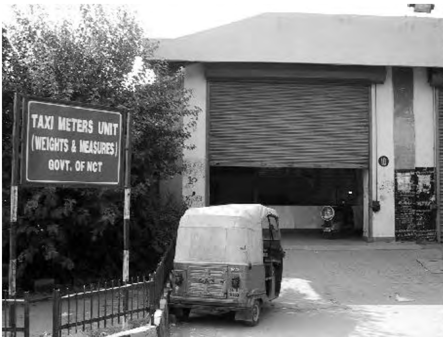
The Taxi Meters Unit, Burari. Why aren't meters working?
