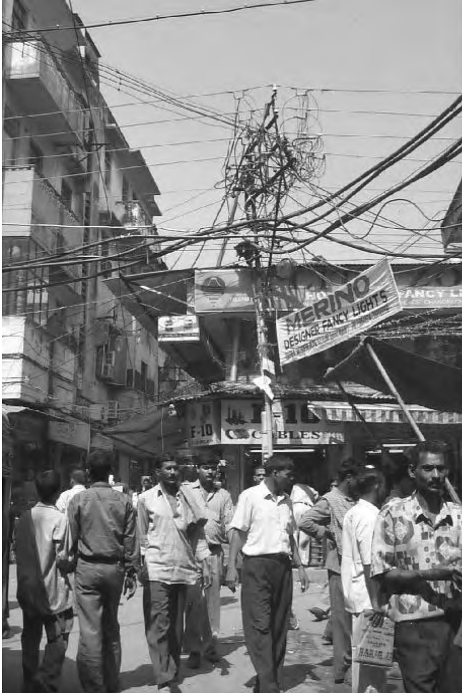
Mangled wires, mangled lives.
